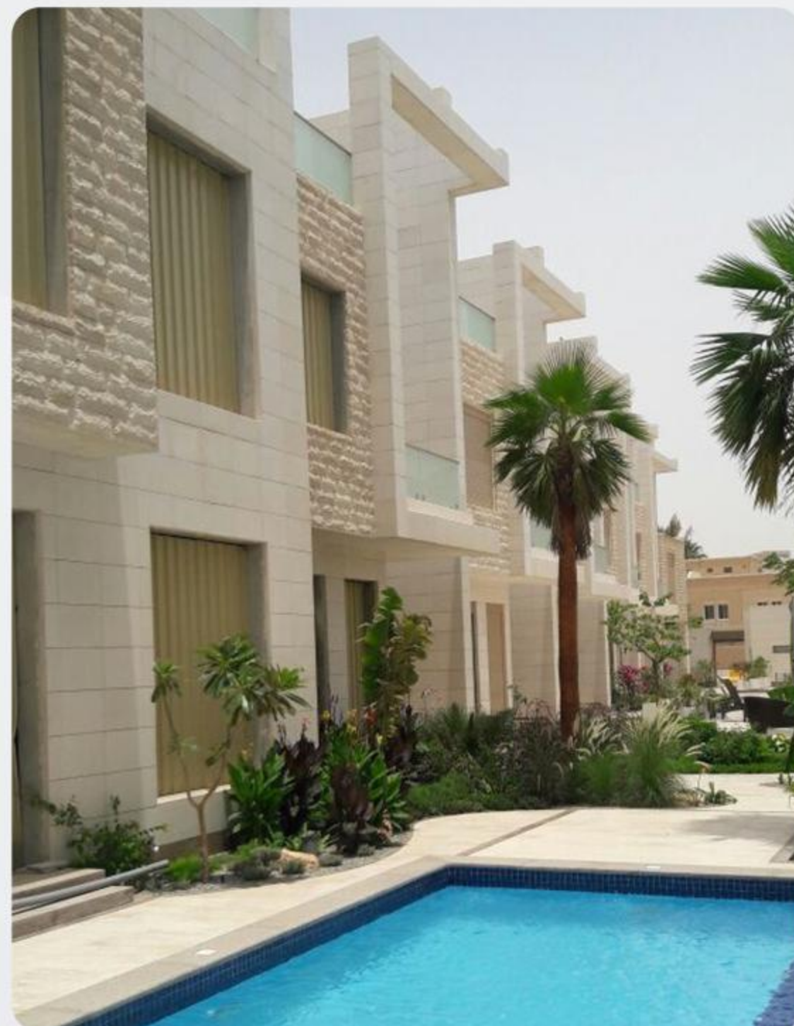
Supply and installation of natural stone for the Al-Khuzami residential complex project 20 villas - Al - Ghazawi Trading Company -Al-Khuzama District- Riyadh
