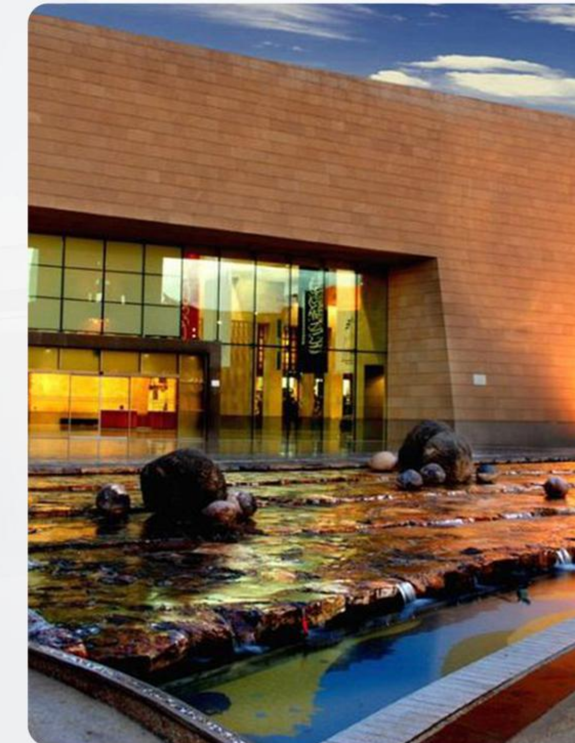
Supply and installation of natural stone for the expansion of the King Abdul Aziz Historical Center Al-Murabba' District - Riyadh
