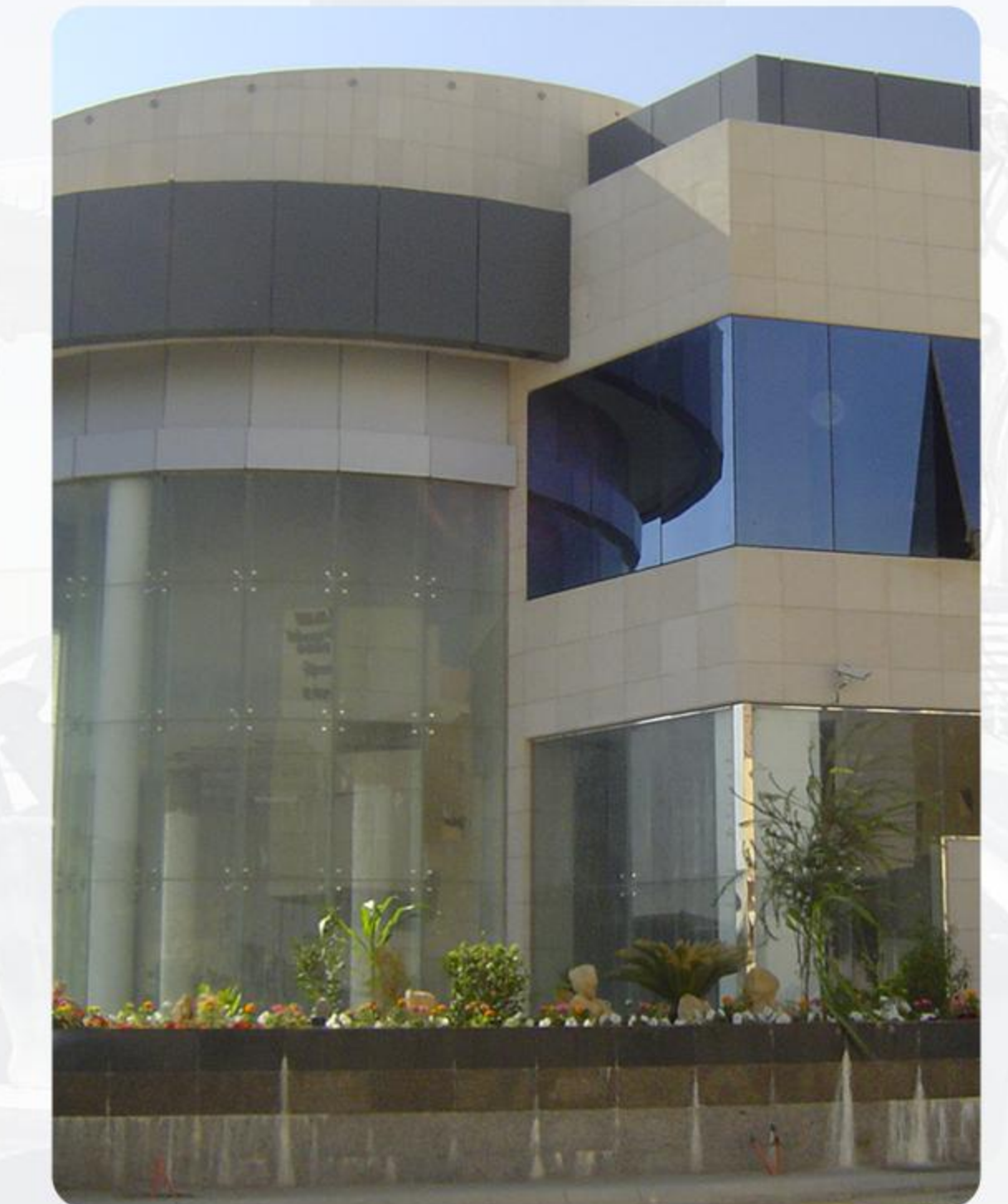
Supply and installation of natural stone for the ministry of Finance buildings project – Al - Arini Contracting Company Hafr Al Batin
