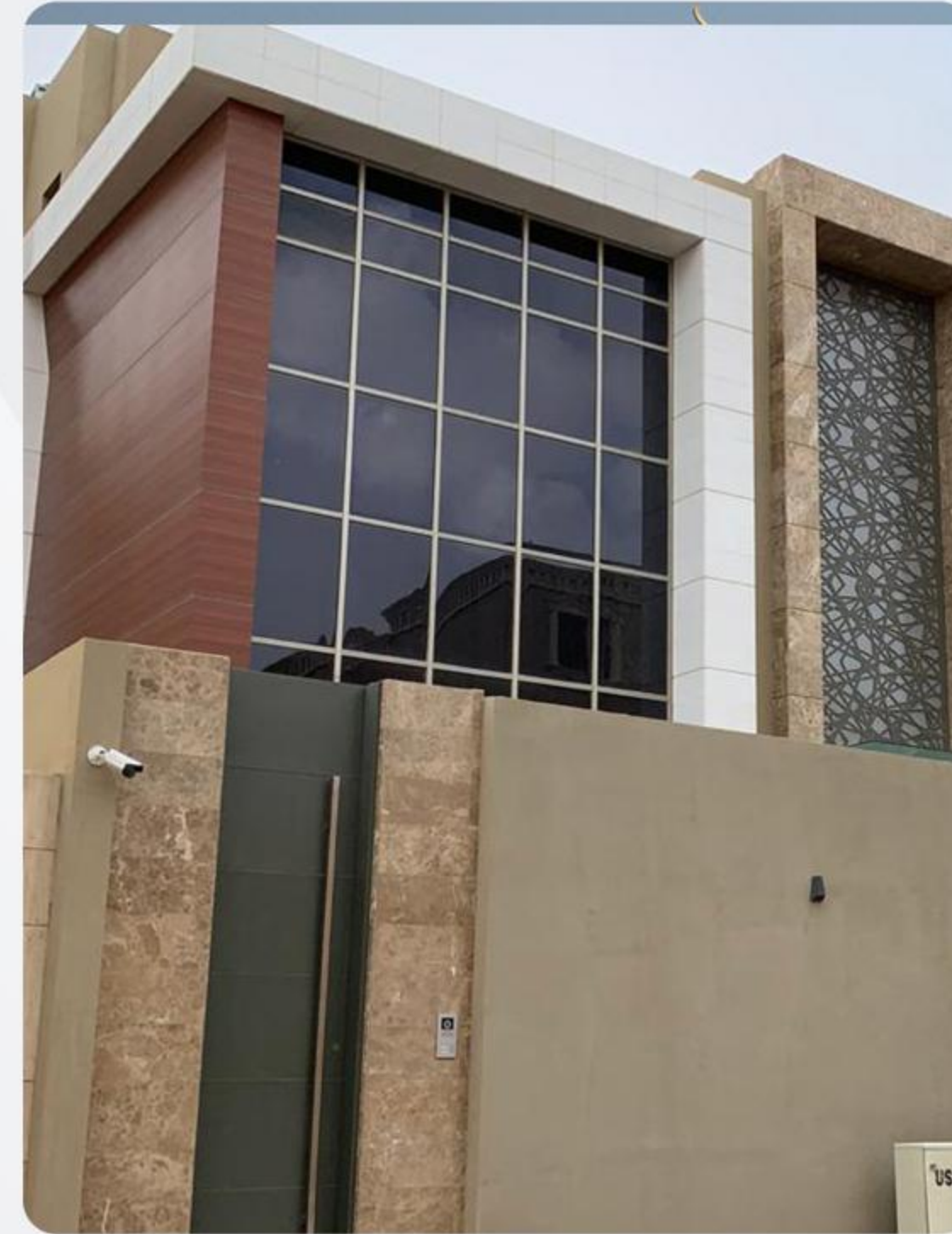
Supply and installation of natural stone villas and palaces for Al - Kreidis Real Estate Company - Riyadh
