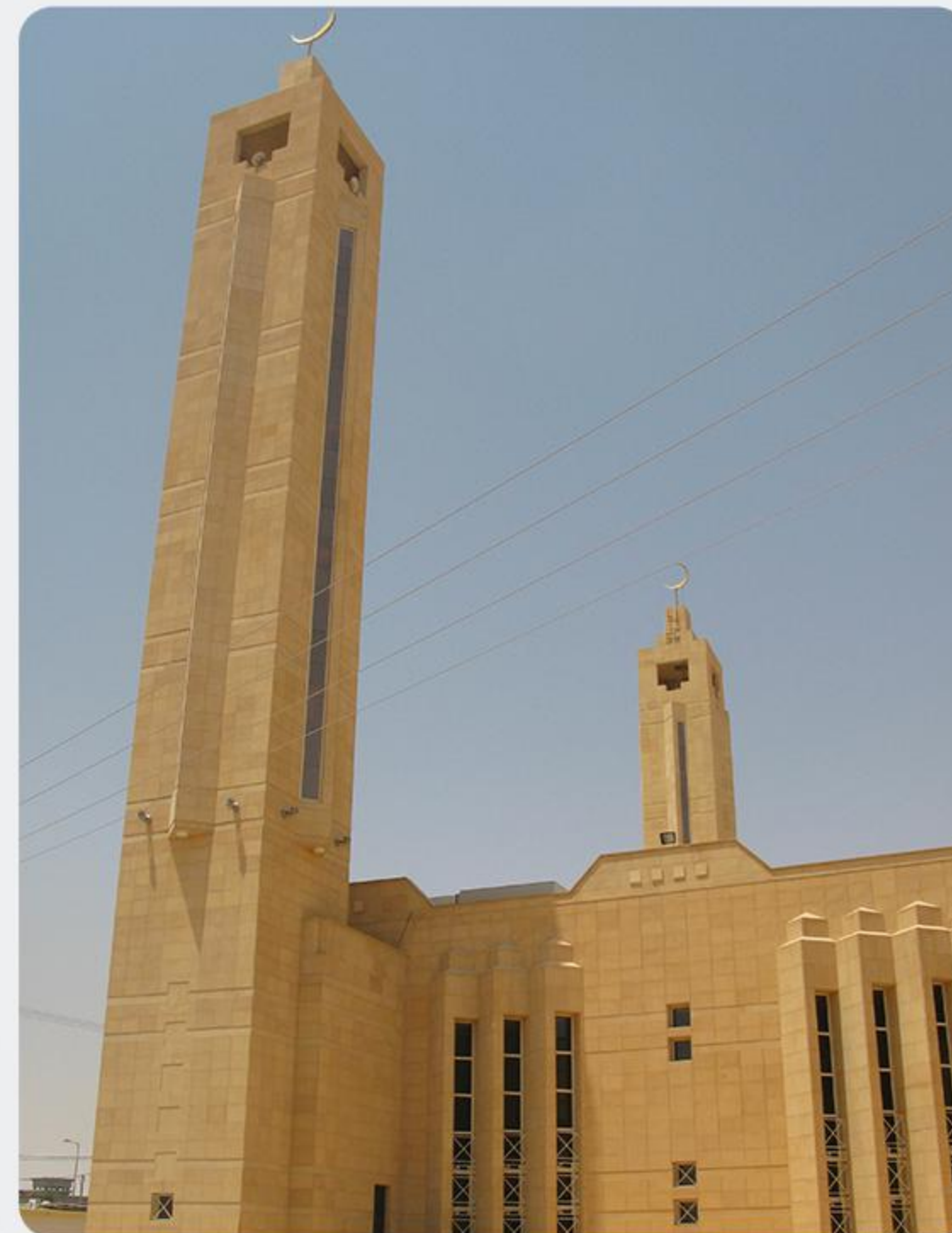
Supply and installation of natural stone, Sheikh Rashid Bin Khaneen Mosque – Al Kharj – Al Dalam
