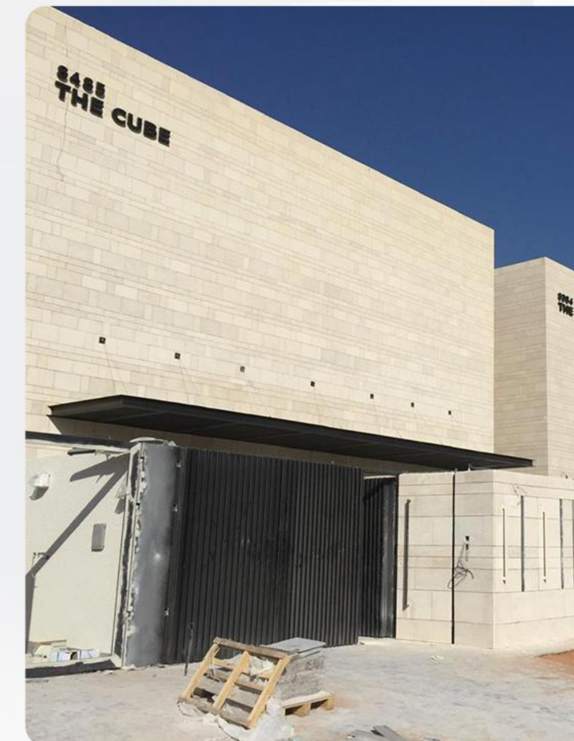
Supply and installation of natural stone for a residential complex project of 28 villas , Al-Rajhi Company for Trade and Industry - Al-Malqa district - Riyadh
