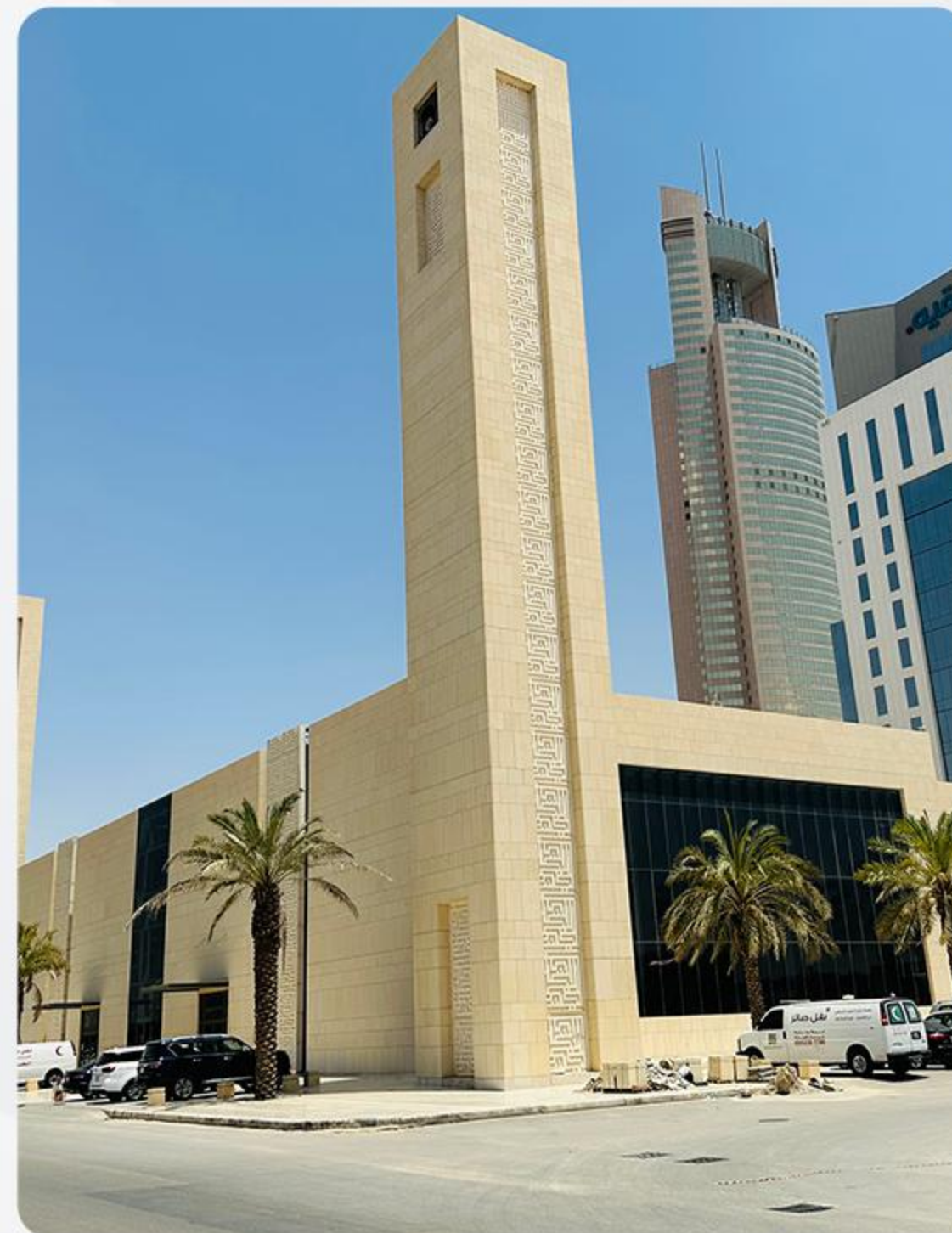
Supply and installation of natural stone , Al - Babtain , Mosque Al - Sahafa District , Riyadh
