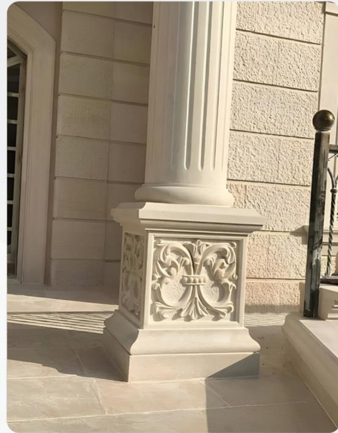
Cladding the columns
